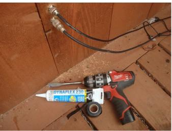
For now a 2m/440 antenna was attached to one connector and a G5RV jr (40m-6m) to the other. Silicon tape was used to seal the connectors because it is easy to remove for future antenna projects.
